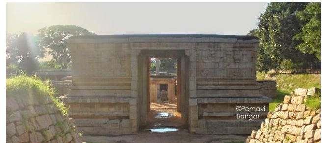
Figure 7: Base of Gopuram of Underground Shiva Temple
