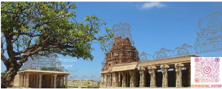
Figure 19: Vijaya Vittala Temple Complex
