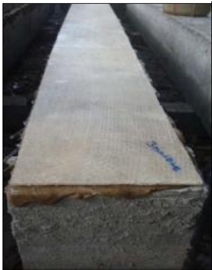
Figure -4: Placing of Laminate over the Beam Soffit
