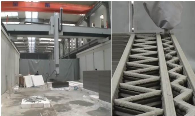
Fig -3: Internal reinforcement of 3DP
