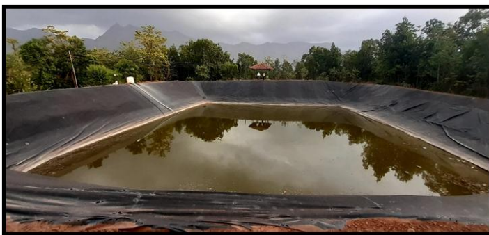
Figure No. 6- On-Site Image of Existing Farm Pond
