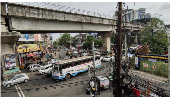
Figure - 3 : Ernakulam - Kaloor Junction
