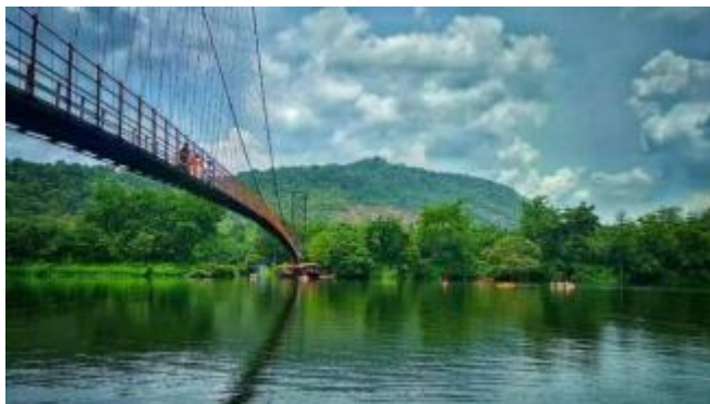
Fig - 2: Inchathotty Suspension Bridge
